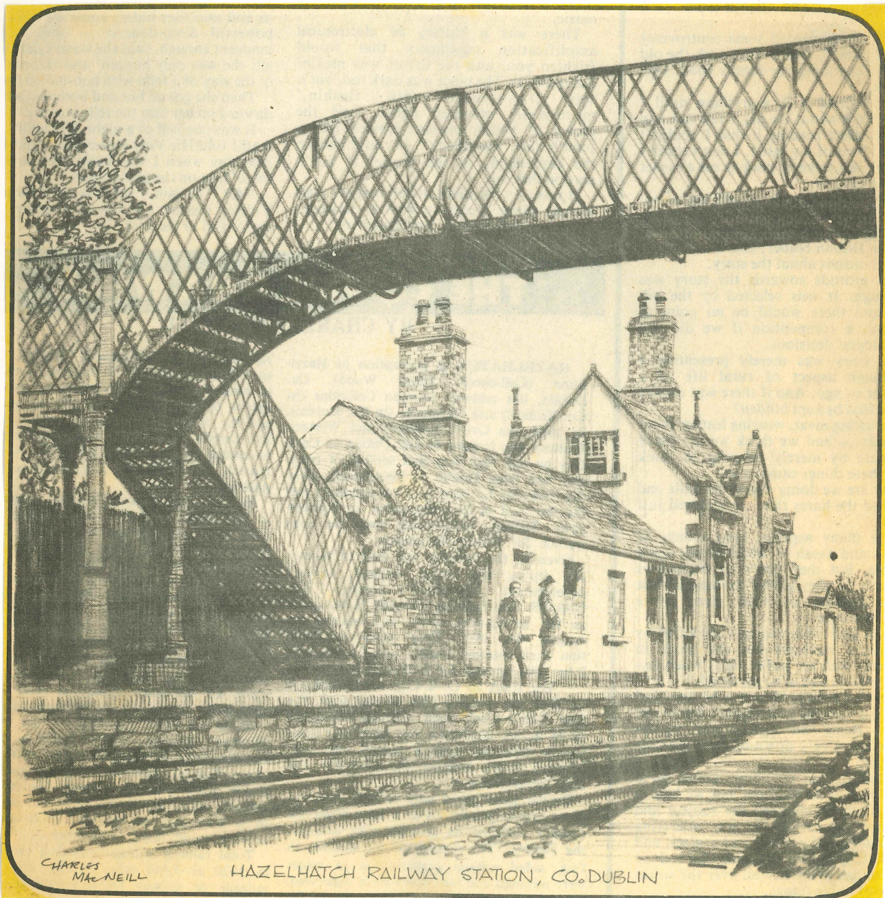
Hazelhatch Railway Station, Co. Dublin, as it used to be.
