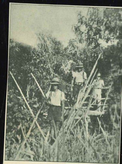
Crossing a Bridge through the Jungle to Debak.
